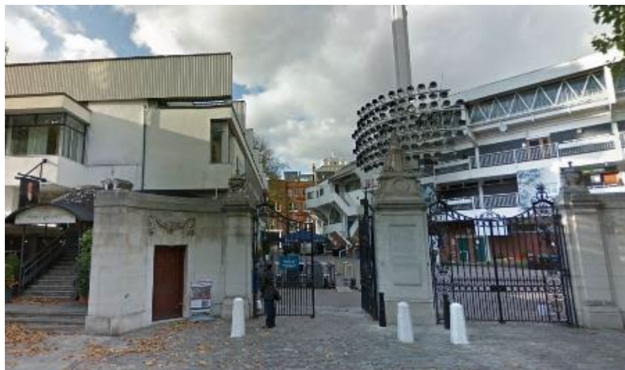
Allen Stand from St John's Wood Road (photo from Google Street View)
