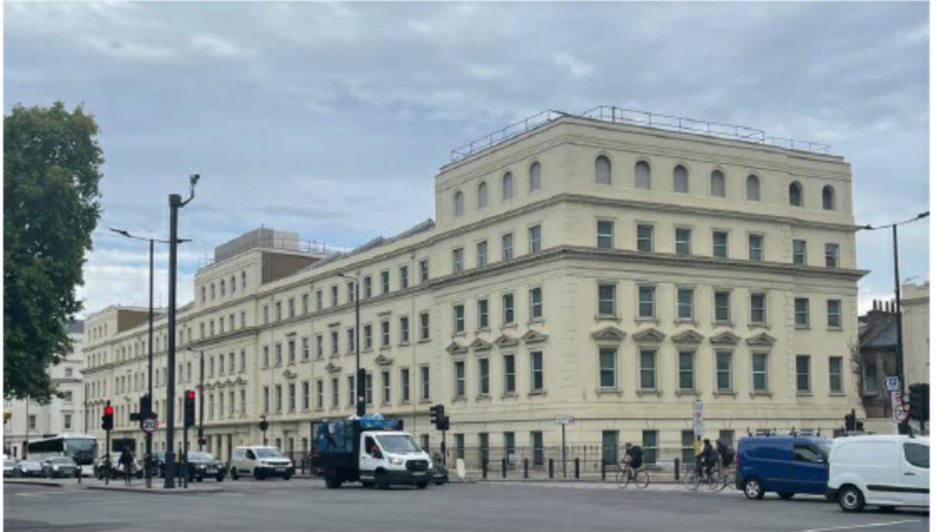
Existing Bessborough Gardens Frontage to Vauxhall Bridge Road
